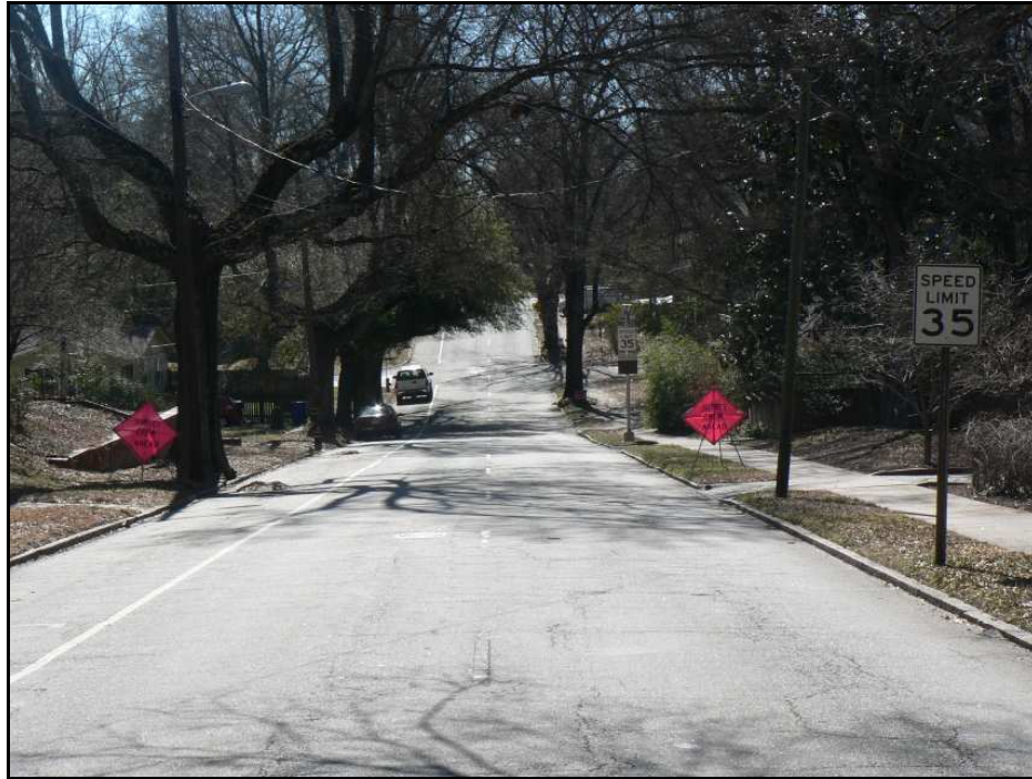
Gregson Street – Showing Roadway Geometrics
